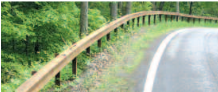
Recommended box beam guiderail.
