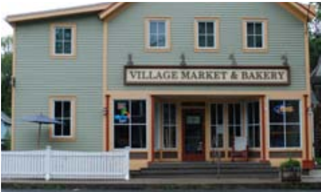
This highly legible sign is perfectly designed to match the character of the building facade, and downlighting prevents glare and light pollution.
