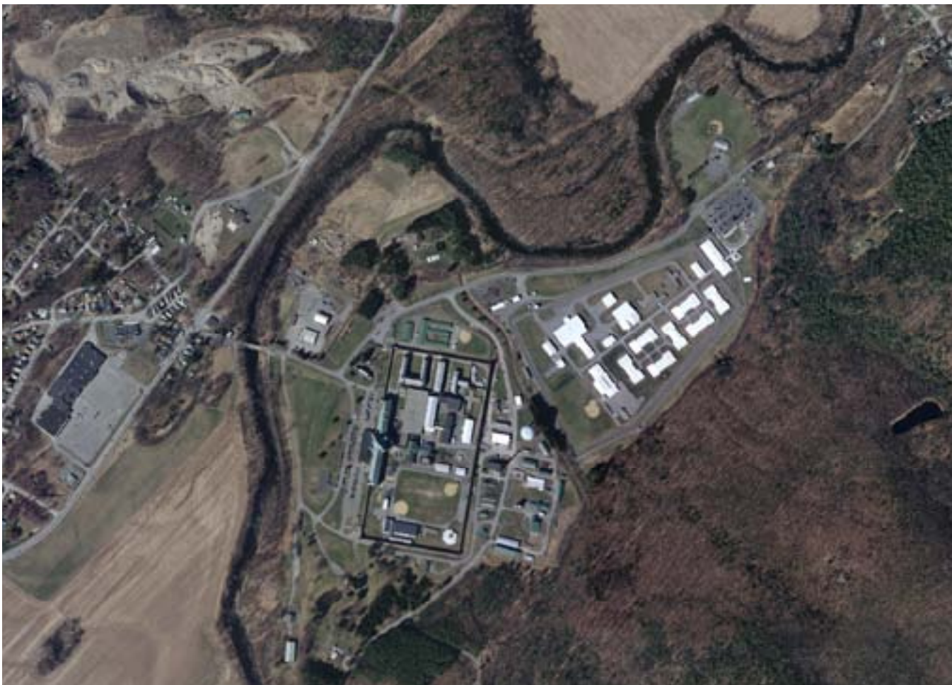
This correctional center complex in Wawarsing is surrounded by vast expanses of undeveloped open space.
