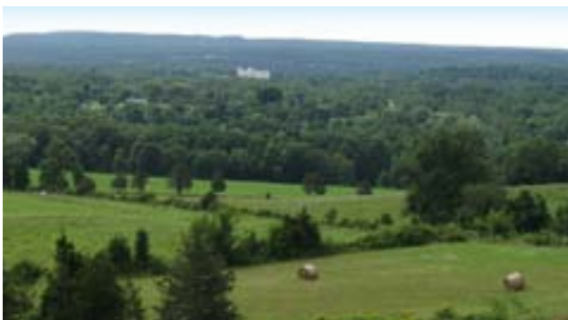
The high-profile siting and contrasting color of this building creates a visual disruption in the landscape.
