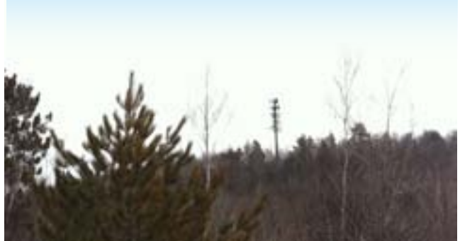
This cell tower made to look like a pine tree employs a common method for blending a necessary utility into the landscape. While it is still noticeable from this angle, its low profile helps to blend it further into the landscape.
