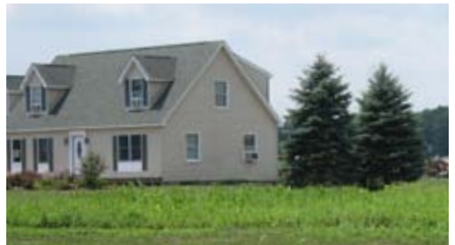
Evergreen trees provide a buffer from winter winds and enhance aesthetics.
